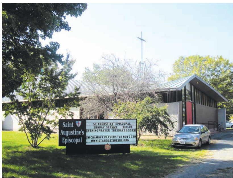
St. Augustine's will remain at the prominent corner of 6th Street, SW and Maine Avenue, SW, but will be housed in a new building on the site.
