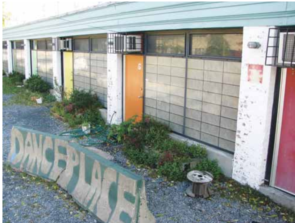
The Brookland Studios adjoining Dance Place will be demolished to make way for the new Artspace project. Photo: Hunter Gorinson.
